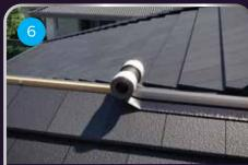
Roll out the **RapidRidge Ridge Flashing** ensuring there is 75mm cover each side of the top course of tiles and on any overlaps.
