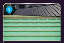
Fix the ridge batten into the **RapidRidge Batten Holder** and lay the tiles as normal across the whole roof.
