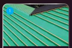
Install the sarking and battens as normal across the roof except the two battens closest to the top. When laying the sarking ensure to leave a sufficient sag (not more than 40mm) to facilitate drainage between each roof truss.
