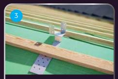
Fix the RapidRidge Batten Holder onto every 2nd roof truss across the ridge and hips, the batten holder can be split or bent to shape as required. Next fix the last two battens at the top of the roof.
