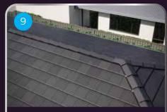
Repeat all the way along the ridge line to the abutment, hip or gable. Apex fixing will require a pre-drilled hole to fix along with clips on other join points. Use a suitable length (depending on roof profile in use) corrosion resistant roof screw with rubber washer to seal.
