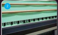
At the eaves around the roof perimeter, fix the **RapidRidge Eaves Vent** to facilitate the air flow under the roof tiles. This will sit on top of the sarking to facilitate drainage.
