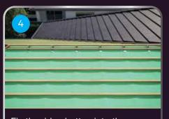
Fix the ridge batten into the **RapidRidge Batten Holder** and lay the tiles as normal across the whole roof.
