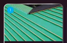
Install the sarking and battens as normal across the roof except the two battens closest to the top. When laying the sarking ensure to leave a sufficient sag (not more than 40mm) to facilitate drainage between each roof truss.
