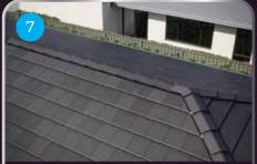
Repeat all the way along the ridge line to the abutment, hip or gable. Apex fixing will require a pre-drilled hole to fix along with clips on other join points. Use a suitable length (depending on roof profile in use) corrosion resistant roof screw with rubber washer to seal.
