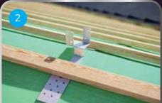
Fix the RapidRidge Batten Holder onto every 2nd roof truss across the ridge and hips, the batten holder can be split or bent to shape as required. Next fix the last two battens at the top of the roof.
