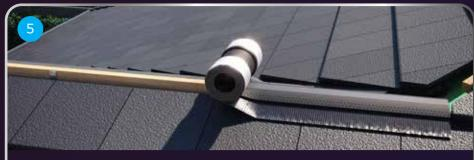
Roll out the **RapidRidge Ridge Flashing** ensuring there is 75mm cover each side of the top course of tiles and on any overlaps.
